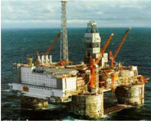
Fig.1-2 Heidrun, concrete TLP
