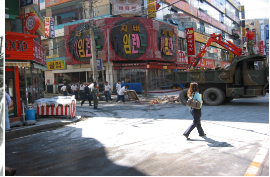
Photo. 1.2 Damaged area by typhoon Maemi in Masan.
