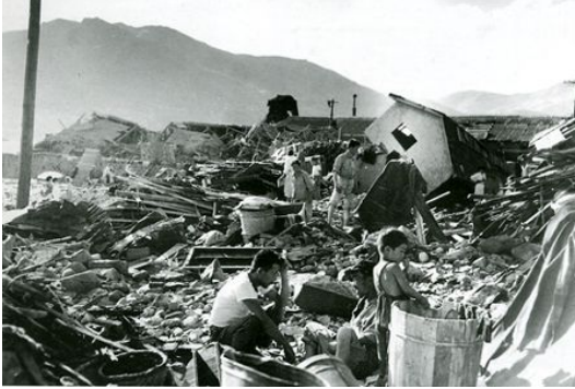
Photo. 1.1 Damaged area by typhoon Sarah in Busan.
