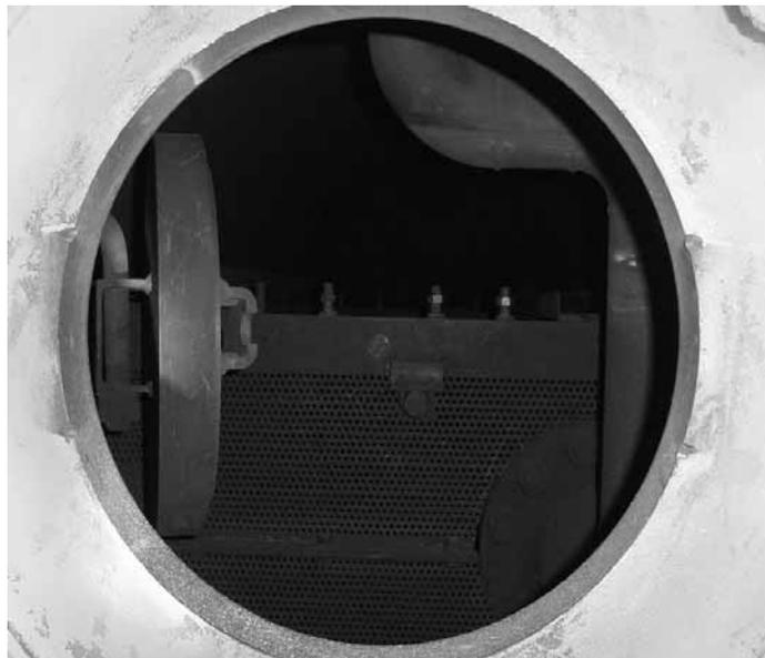
Fig. 1.7 Inter-fitted de-superheater in the water drum of Main boiler
