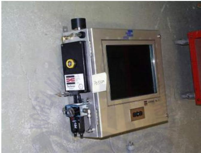
Fig. 2.3 Photo of pressurized enclosure
