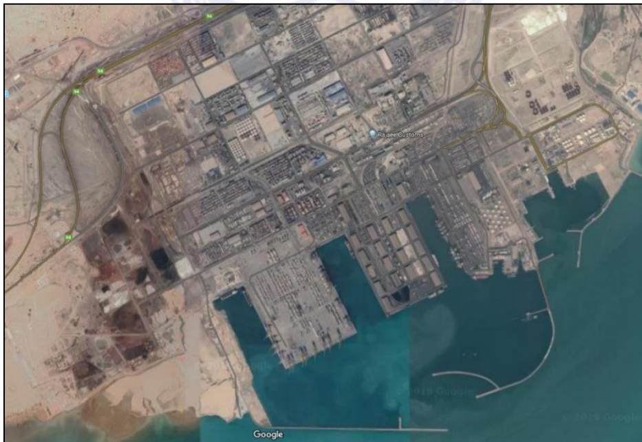
Figure 4.2. Shahid Rajaei port overview Source: www. PMO.ir
