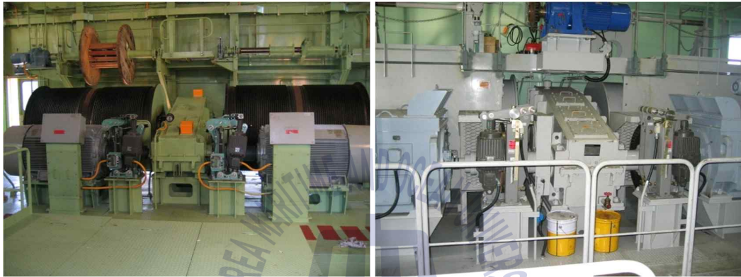
Fig. 2.6 Hoist unit of the STS crane
