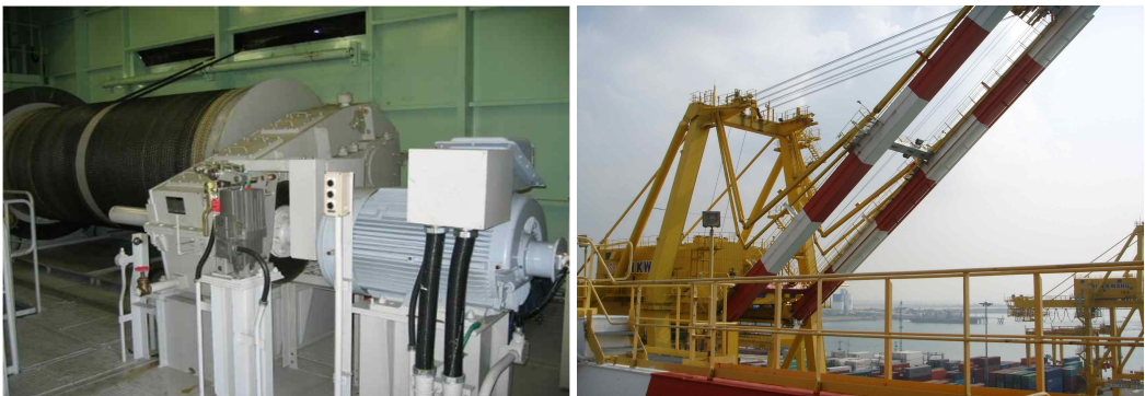
Fig. 2.9 Boom hoist device of the STS crane
