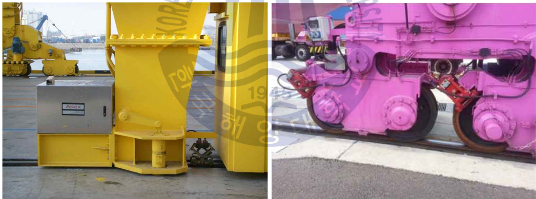
Fig. 2.13 Rail clamp of rail clamping type(left) & wheel brake type(right)
