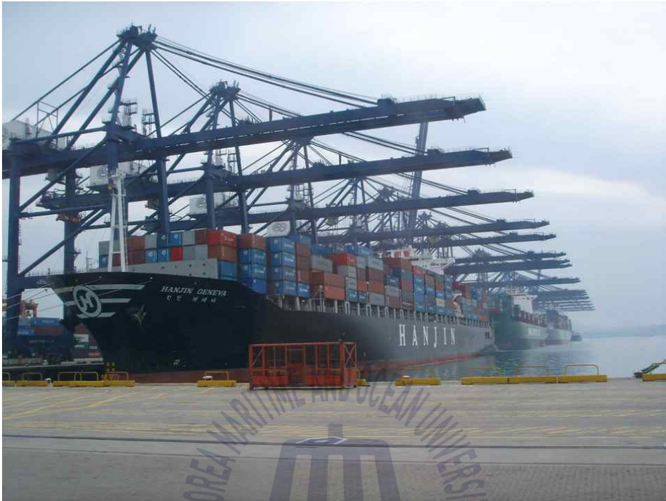
Fig. 2.4 STS crane & container ship
