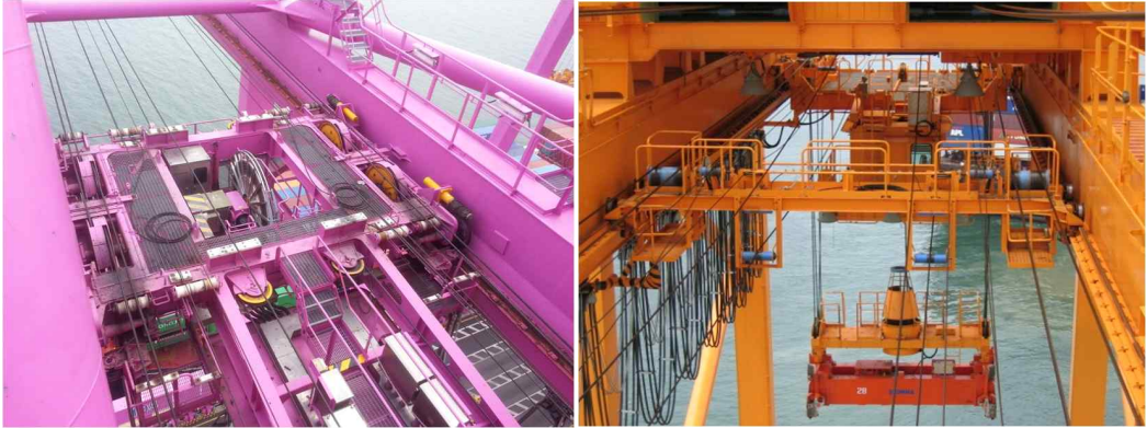
Fig. 2.14 Trolley of the port crane
