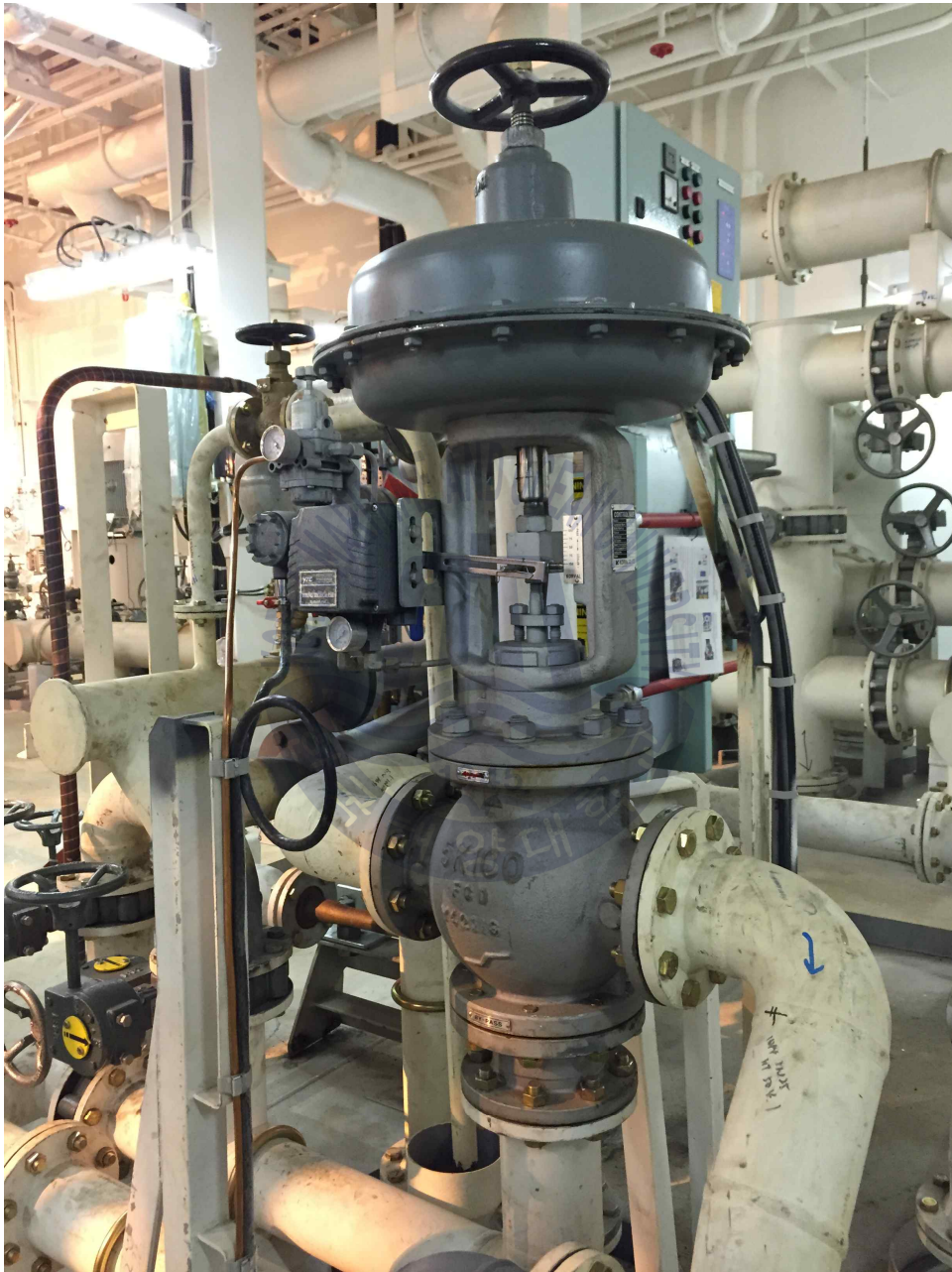
Photo 2.1 Pneumatic 3-way control valve with valve positioner and I/P converter
