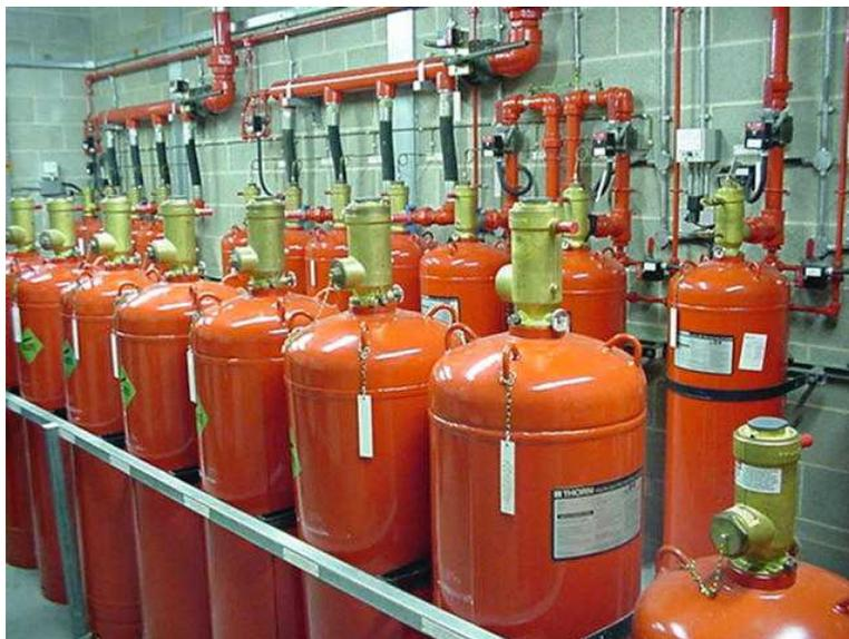
Fig. 26 Installation of banked design
