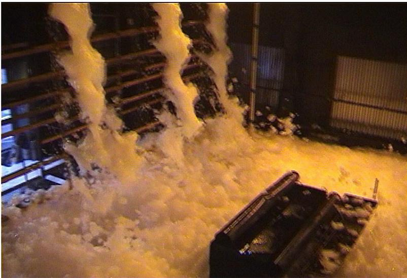
Fig. 2 Picture of high expansion foam system flooding
